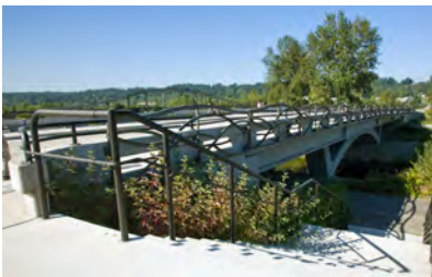
Cliff Garten. Sammamish, WA
