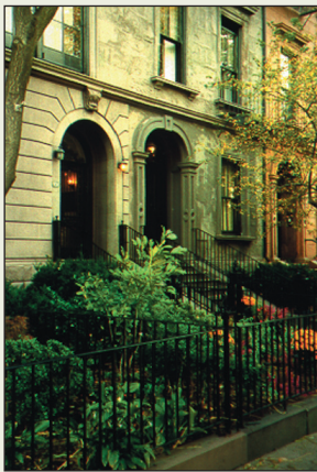
Individual residential unit entrances and enough setback to allow a smooth transition from public to private space lend a sense of beauty and “human-ness” to the street.
