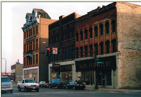
The North Quadrant has strong edges, such as this row of historic commercial buildings on the south side of East 7th Street.
