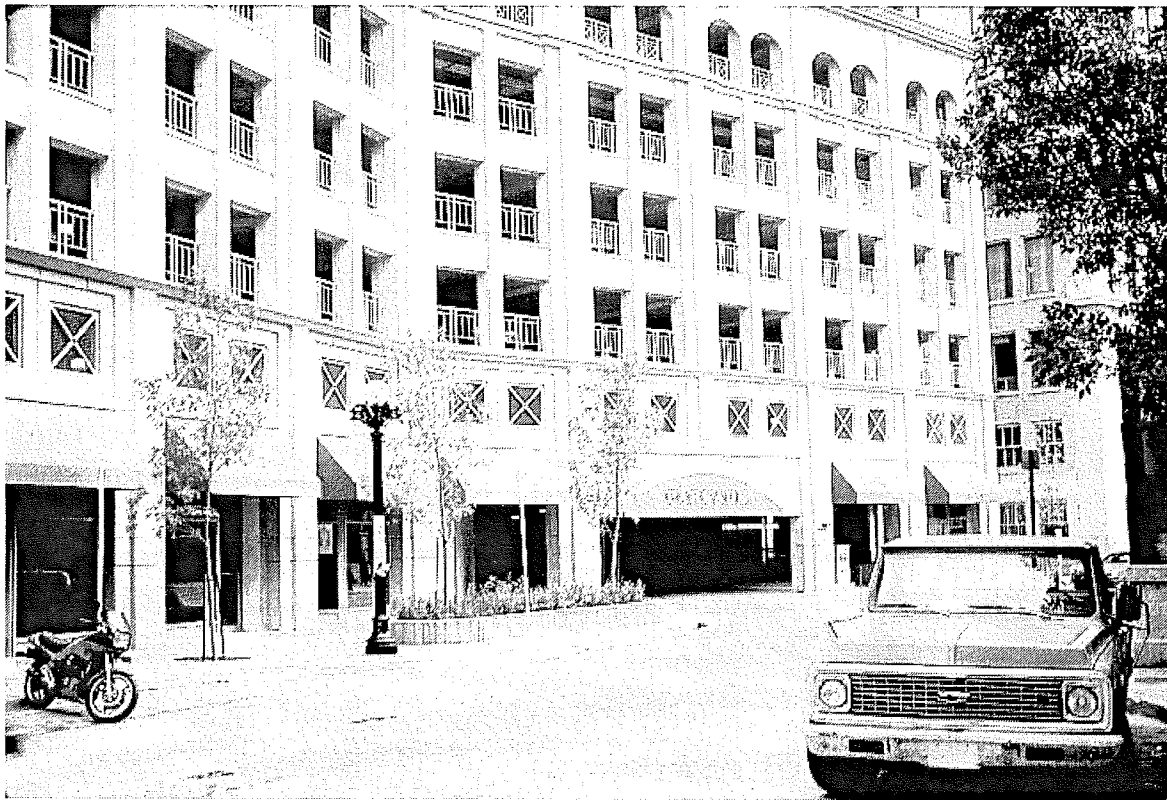
This structure has the appearance of a typical commercial building rather than a parking ramp. The punched openings at the parking levels relate to the window proportions of surrounding buildings.
